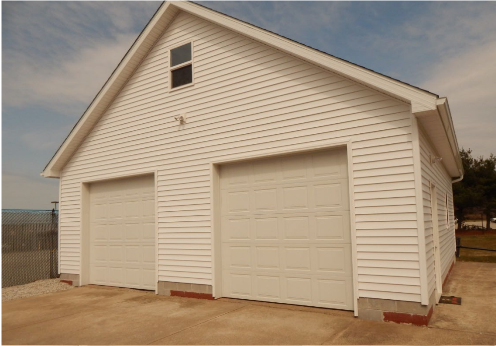
Garage with block foundation
