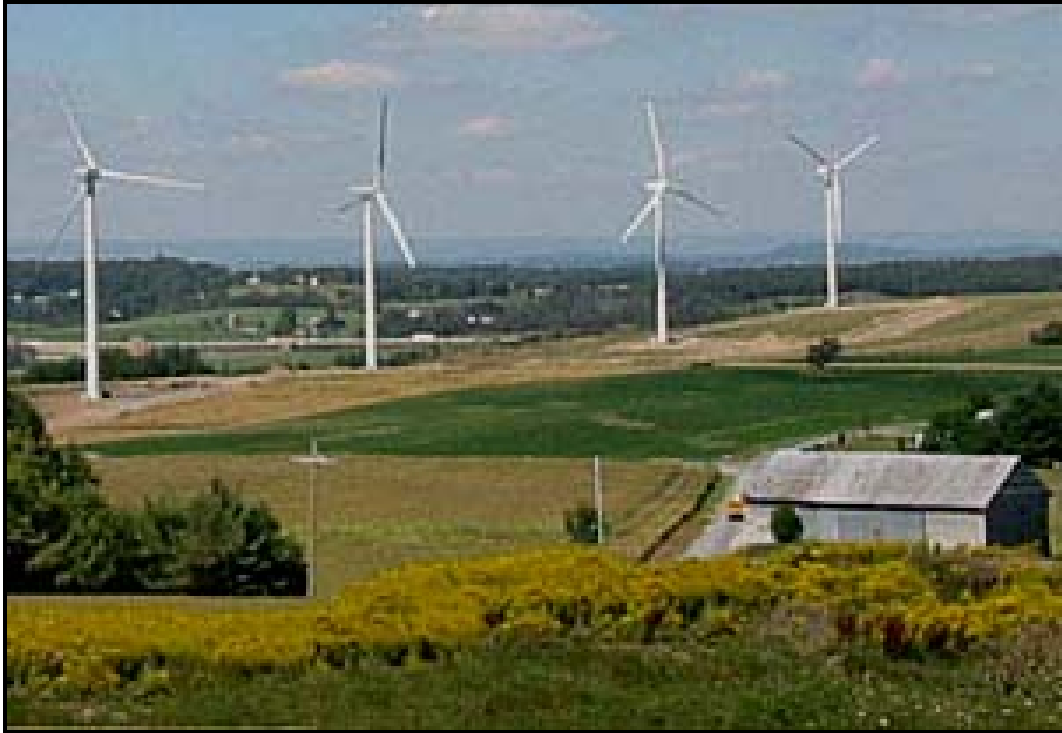
Photograph of Mill Run wind farm located in Fayette County. Taken from website of The Reinvestment Fund ( http://www.trfund.com/financing/millrun2.htm )
